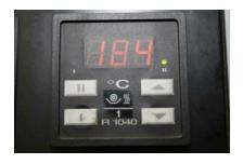
Temperature setting (melting equipment) in line with recommendation of hotmelt supplier (please check Technical Data Sheet)
